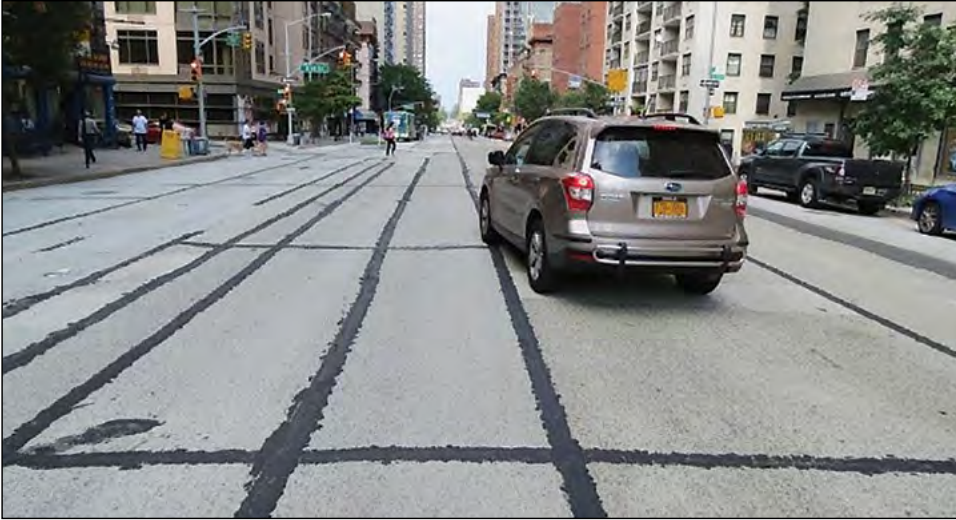
FIGURE 2 First Avenue milled, sealed, patched, and ready for overlay.
