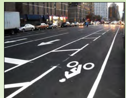
FIGURE 4 Completed First Avenue project.
