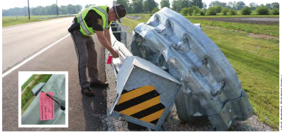
Law enforcement official applying damage tag to infrastructure damaged by motor vehicle crash.
